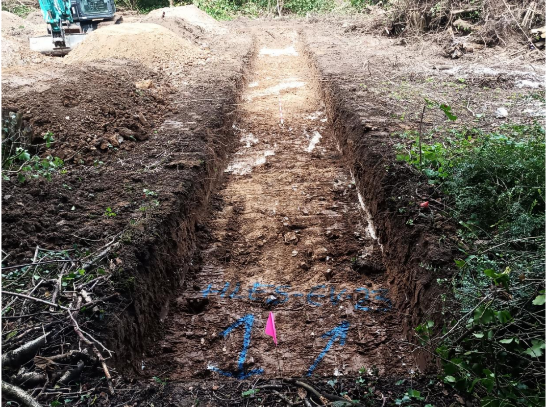
Plate 1 Trench 1, viewed from the southeast
